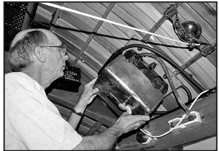
Tom Peyton installing the breaker. – Two photos © 2008 Darrell Arndt.
